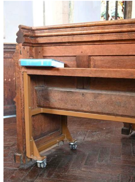
Example of metal frame fixed to pews
